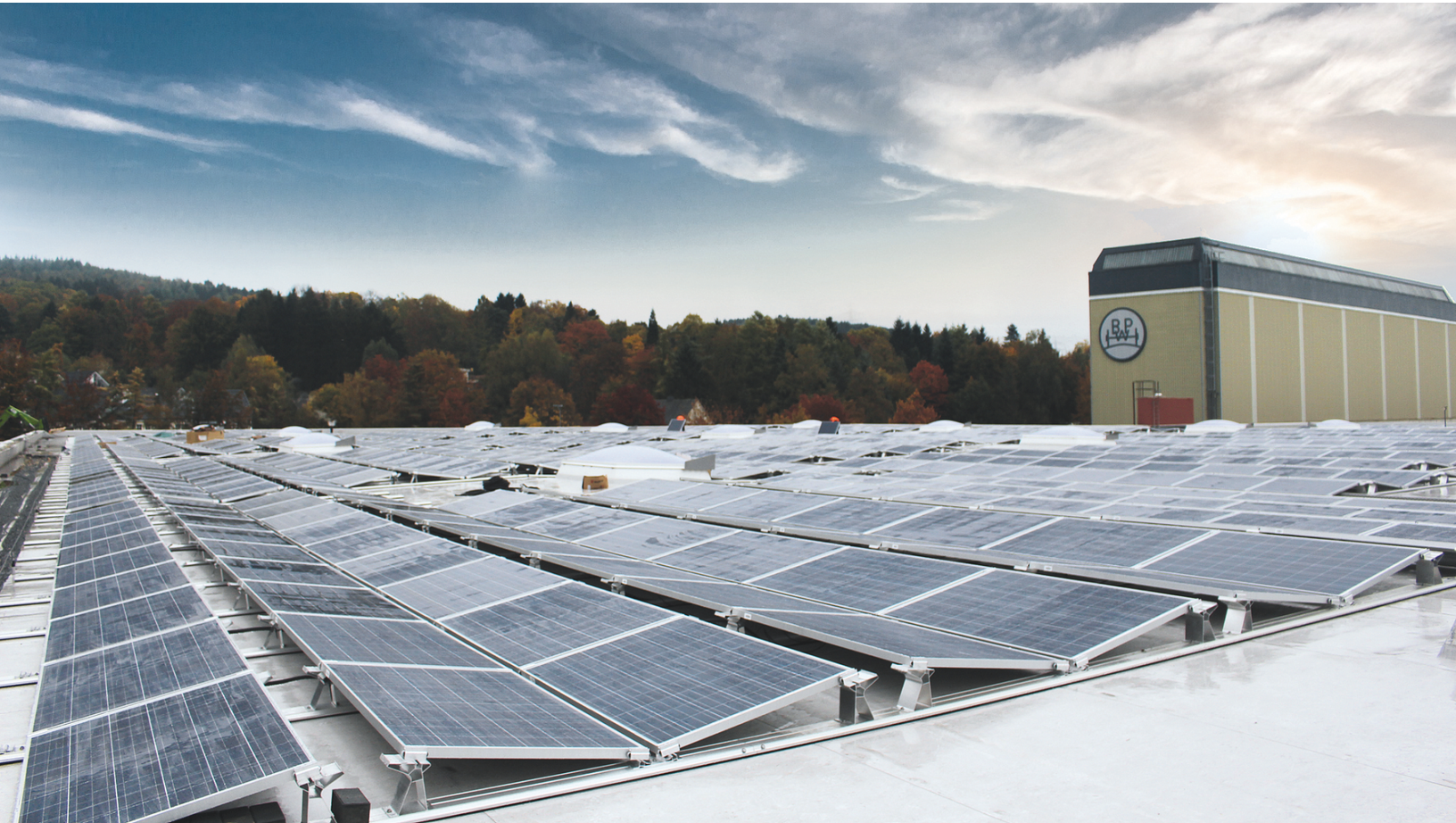
A factory roof at the works in Wiehl accommodates a 3,100-sqm photovoltaic system.
